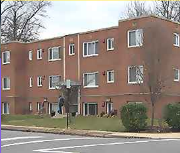
Mt. Vernon Ave., Alexandria / Adams Apartments
