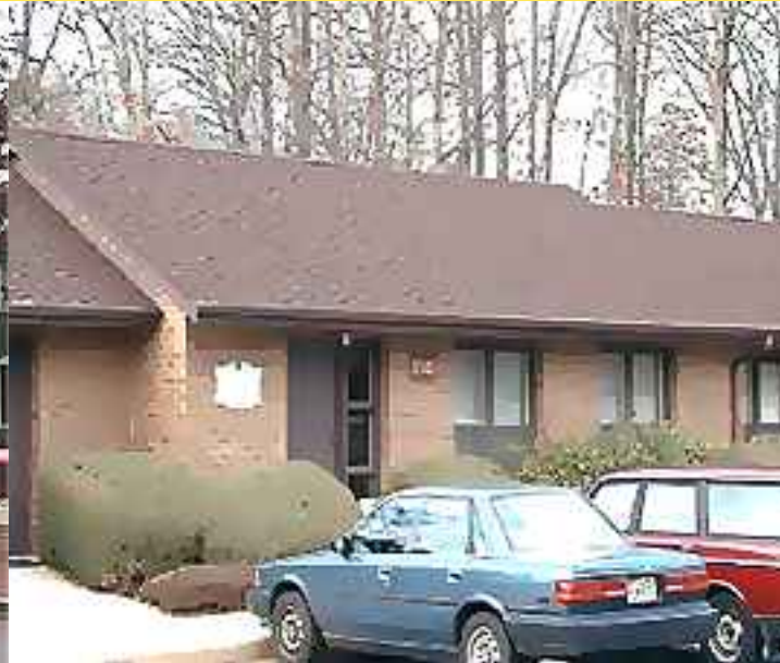
8340 Traford Ln., Springfield / Professional Park
