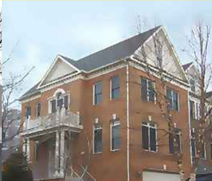
132 Rees Place, Falls Church / Rees Estate
